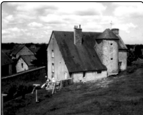
The Leroux Manoir house and outbuildings, seen here in 1997, are just as they were in 1944. The blown-out wall near the front door has been repaired.
